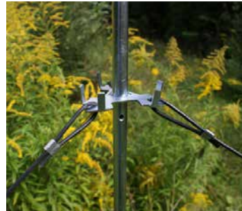
...Hook the three slot traps to the hooks.
